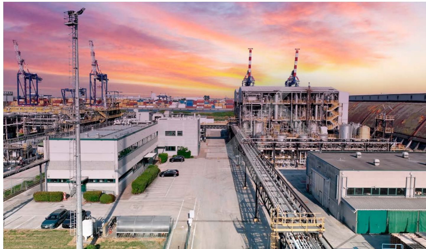
Endura Plant, The Chemical Hub, Ravenna (Italy).
